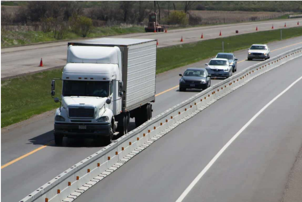
Raised Median with Portable Steel Barrier – Positive Separation
