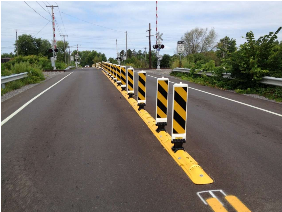
Raised Median with Lane Separator System (curbing with vertical panel delineators)
