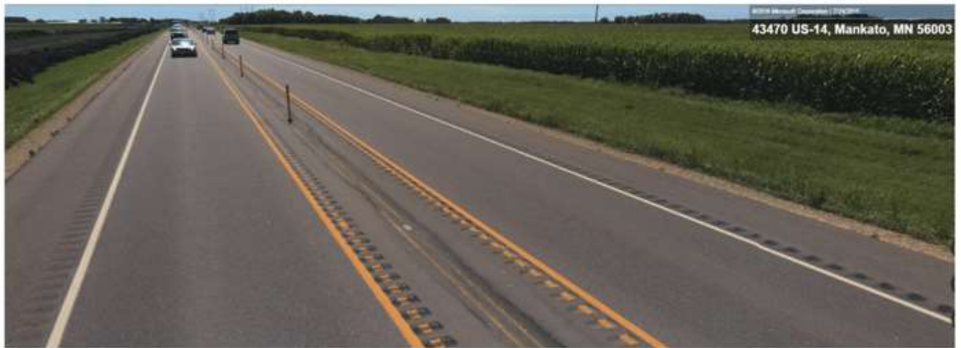
Flush Median with Wide Separation and Rumble Stripes – Include Flexible Delineators
