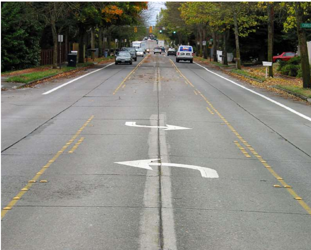
4-Lane Conversion to TWLTL with Left-Turn Pocket developed for Traffic Signal
