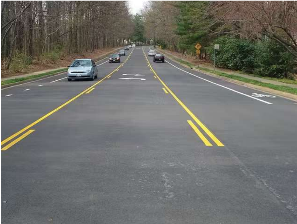
4-Lane Road Diet Conversion to TWLTL and 2-Lanes (w/Bike Accommodation)
