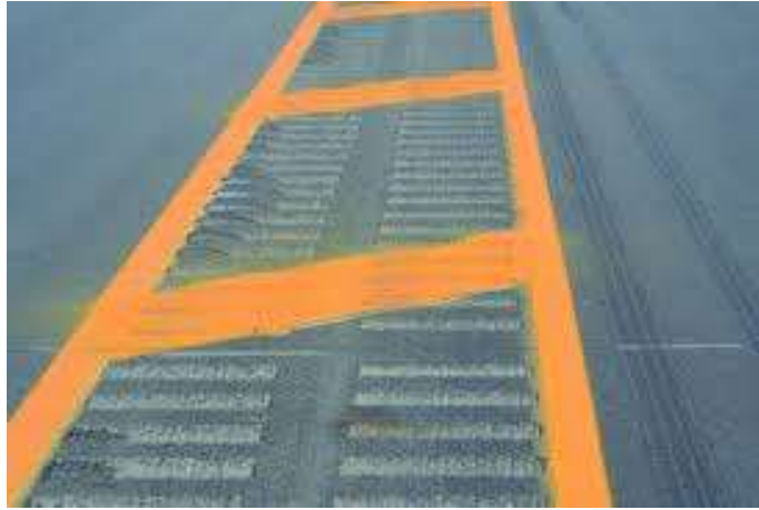
Flush Median with double run of Rumble Strips with Painted Diagonal Crosshatch Markings
