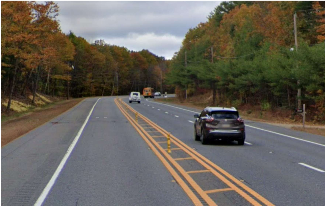
Flush Median with Crosshatching, Rumble Stripes & Flexible Delineators (Route 140, Gardner)
