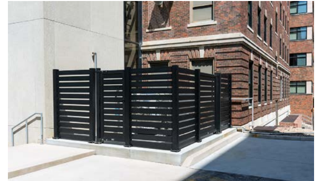
Screening service equipment, image credit: Cityscape inc
