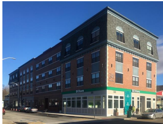
Figure 27. Inappropriate mansard roof design in Beacon, NY. The roof is too tall relative to the floors below. The dormers are inset into the roof instead of projecting from it. The roof projects beyond the wall below. (Gaither Pratt)
