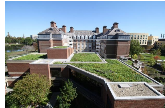
Figure 115. Green roofs can help cool buildings while absorbing stormwater and carbon (recovergreenroofs.com)
