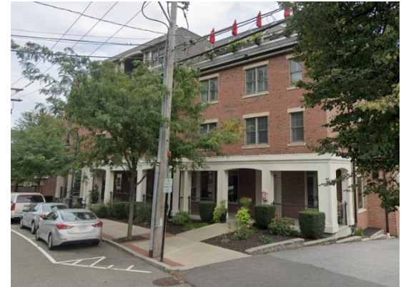
Figure 44. At 36 Central Ave in Milton, an elevated “porch” helps mitigate a grade change along the sidewalk from one end of the building to the other. A sloped walkway leads up to the porch at the end of the building that is closer to the sidewalk grade. This eliminates the need for a less accessible ramp (Google Streetview).
