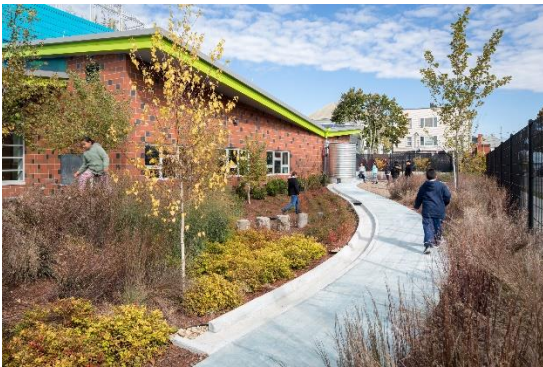
Figure 118. Rain gardens and a cistern at a school in New Bedford. The cistern collects rainwater from the roof. It can be opened to fill the runnel next to the sidewalk. (Dodson & Flinker)
