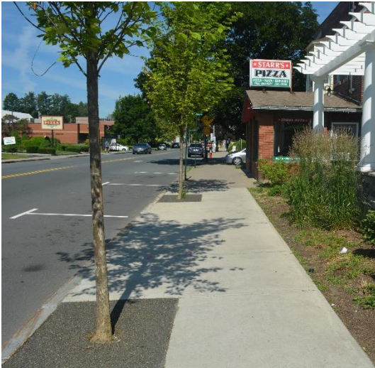
Figure 86. Tree pits can be surfaced with permeable materials, in this case permeable rubber, to allow water and air to reach plant roots, while still providing an accessible surface for pedestrians (Dodson & Flinker)
