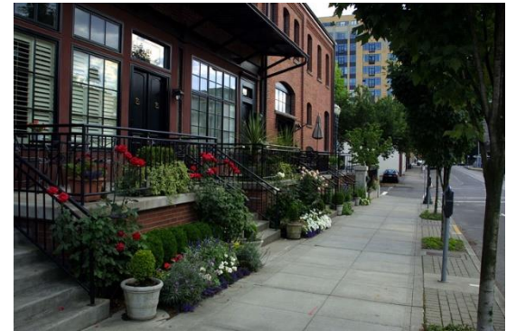
Figure 76. When a retaining wall is unavoidable, attention should be paid to how it relates to both the sidewalk and the building. Here, the retaining wall creates space for a front terrace with seating. A small planting area that is integrated into the design of the protruding steps softens the edge of the retaining wall.
