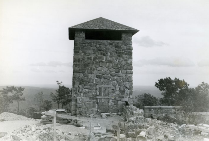
Eliot Tower construction, 1937
